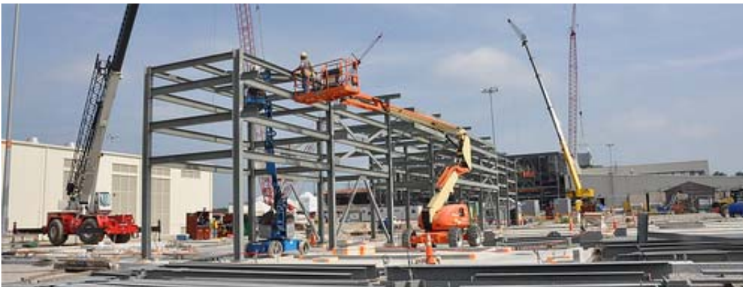
The SCWO processing building joins the MDB and CSB in going vertical
