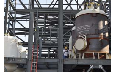
An agent holding tank, agent surge tank, and three spent decontamination fluid tanks are installed at the MDB
